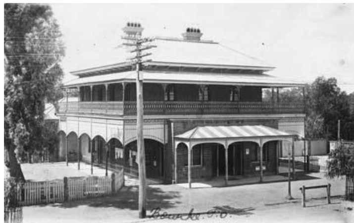
Figure 1. The Stevenson screen (possibly with a copper or iron roof) and anemometer pole occupy a 10 m wide strip that was added to western (right) side of the post office land-title in 1891. (1920 photograph courtesy of the National Library of Australia.) The second storey was added to the original 1880 building in 1889.
